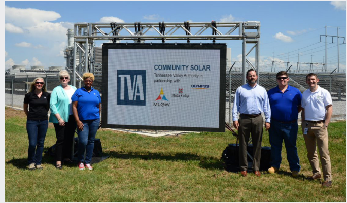
Allen Combined Cycle Plant in Memphis is the most efficient combined cycle plant in the TVA gas fleet and includes more than 3,000 solar panels that provide just under 1 megawatt of renewable energy capacity.
